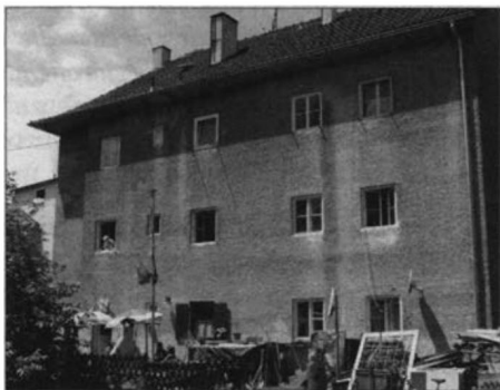
The back of the house at Reichenhaller Strasse 41
